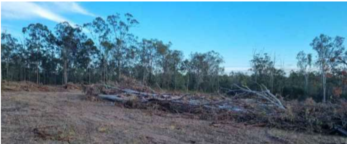
FIGURE 2 - SITE DURING WORKS
